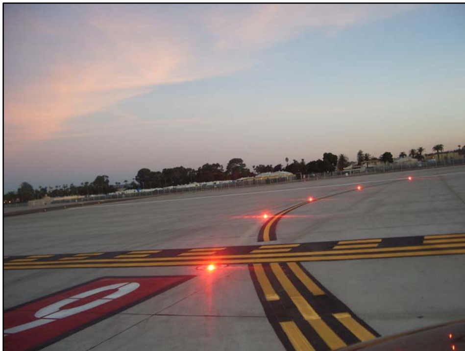
FIG 2-1-10 Runway Entrance Lights
