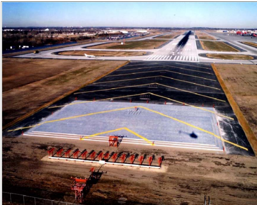
FIG 2-3-42 Engineered Materials Arresting System (EMAS)
